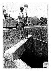
and storm sewer utility networks. GPS field crews conducted comprehensive top-side manhole inspections on sanitary and storm sewer manholes and also GPS located curb stops to integrate into the waterline network.
