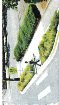
ROADWAY STORMWATER CAPTURE
