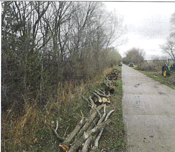
Project 4, Tactic 2: Ten new volunteers cut the larger trees and stacked logs for removal by the community.
