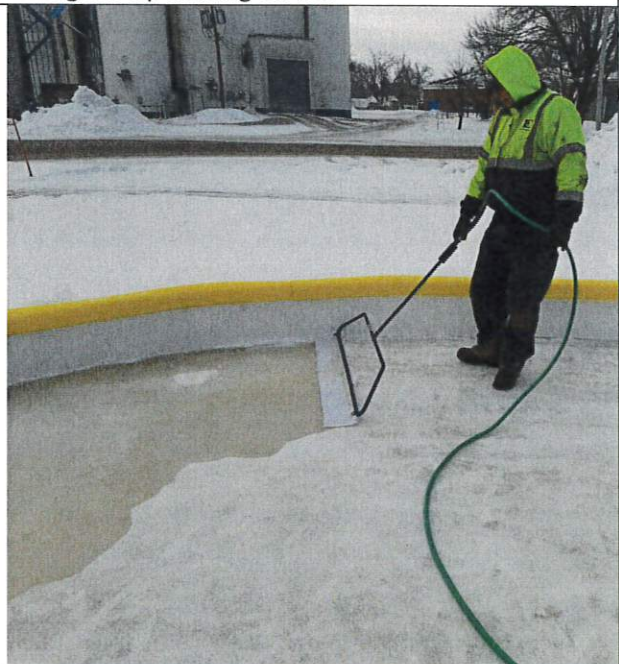
Project 2, Tactic 2: The rink ice was maintained by grooming with a "mini-zamboni" (a perforated tube wrapped in a towel and powered by a garden hose) and a patient worker this year.
