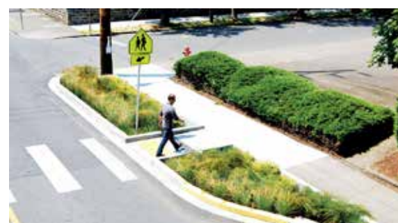
ROADWAY STORMWATER CAPTURE
